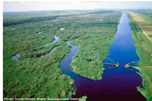
Figure 1 Small dam on the channelized portion of the Kissimmee River in Florida helps to restore wetlands.
